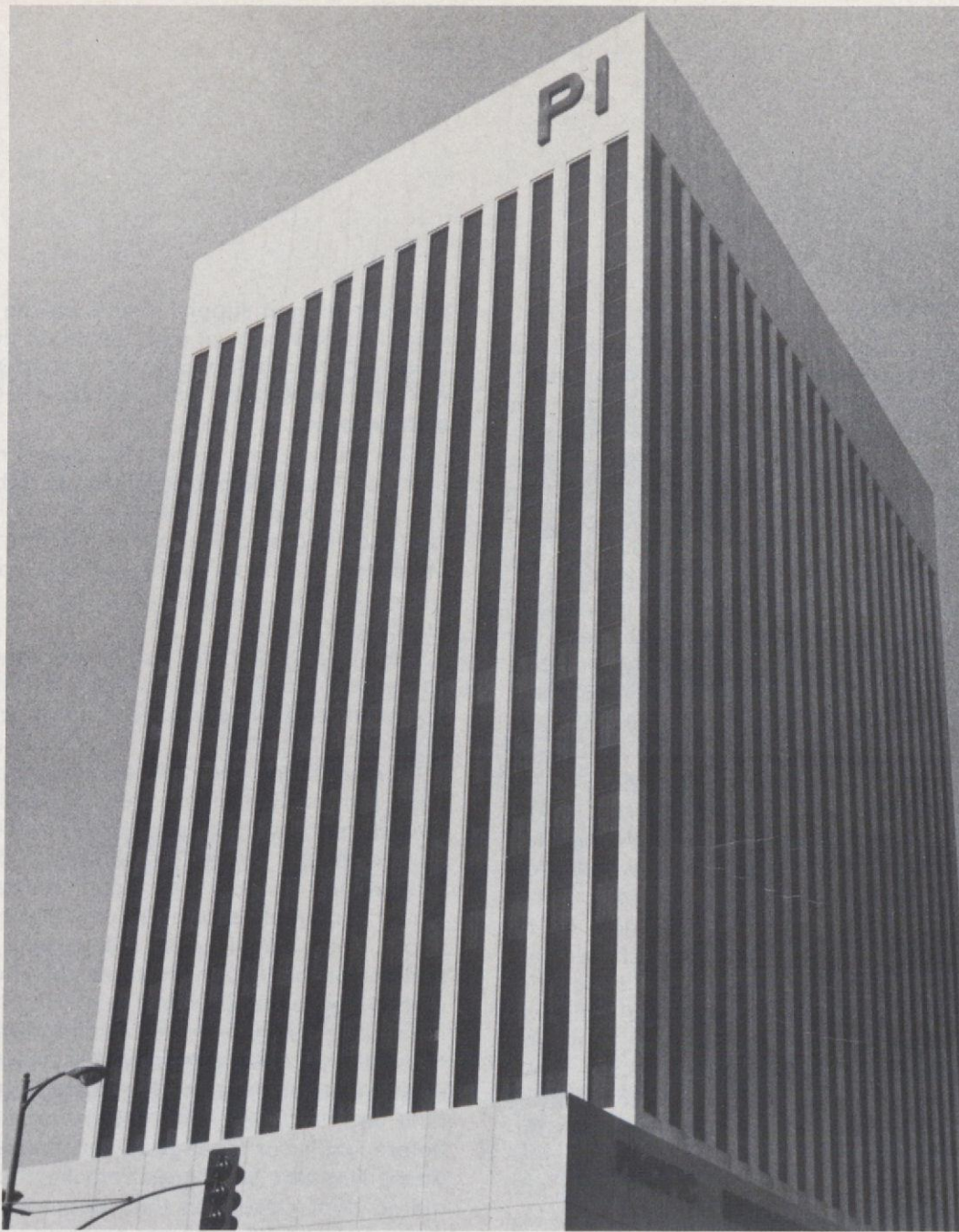
An electronic security and fire detection system will be used in the new, 18-story Pacific Indemnity Building in Los Angeles. The system will allow one guard in the lobby of the building to monitor 160 zones as well as automatically alarming, locking and unlocking all of the stairwell doors.
