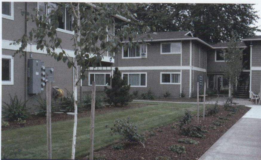
Parkland Terrace, a 52-unit senior housing community, is located just off Ocean Beach Highway in Longview, Wash.
