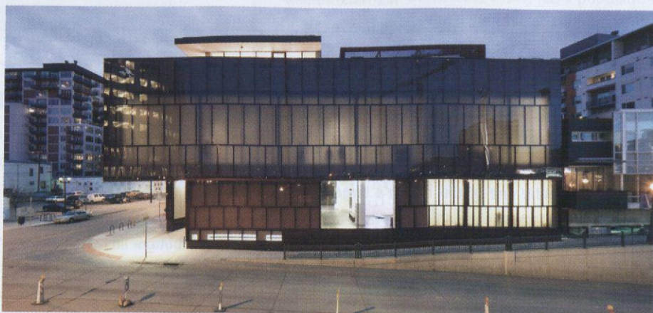
MCA Denver's exterior was partially created with Monopan, a translucent recycled building material.
