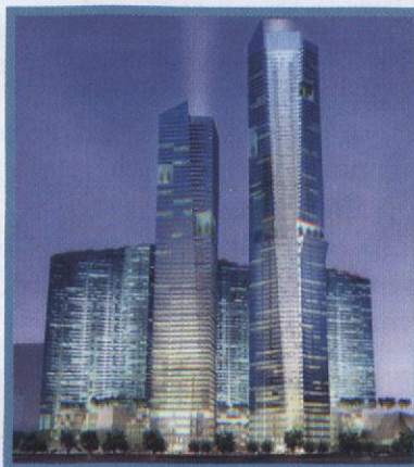
The 70-story Dalian Center Super Tower One in Dalian, China, will stand 1,235 feet, just 15 feet shorter than the Empire State Building.
