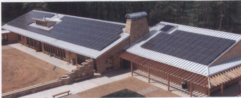
The Aldo Leopold Legacy Center's 198 roof-mounted solar panels produce 50,000 kilowatt hours of energy per year.
