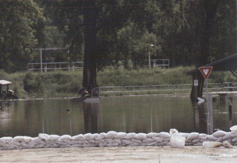
RIVER WATER IN IOWA THREATENS TO FLOOD A RESIDENTIAL STREET.
