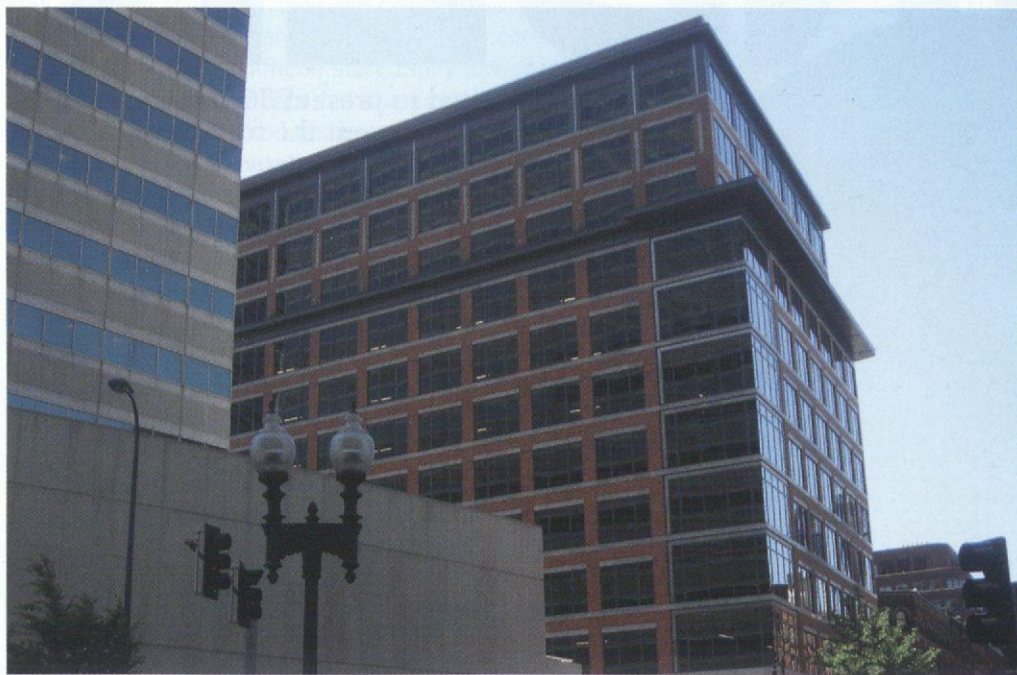
TWO FINANCIAL CENTER IS A MAJOR PROJECT IN BOSTON, ON TRACK FOR COMPLETION IN 2009.
