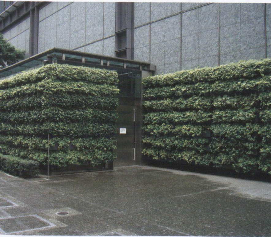
[LEFT] GREEN WALLS BLOCK DIRECT SUNLIGHT AND LOWER TEMPERATURES OF THE INTERIOR AND THE SURROUNDING AREAS OF THE NEW MARUNOUCHI BUILDING IN JAPAN.
