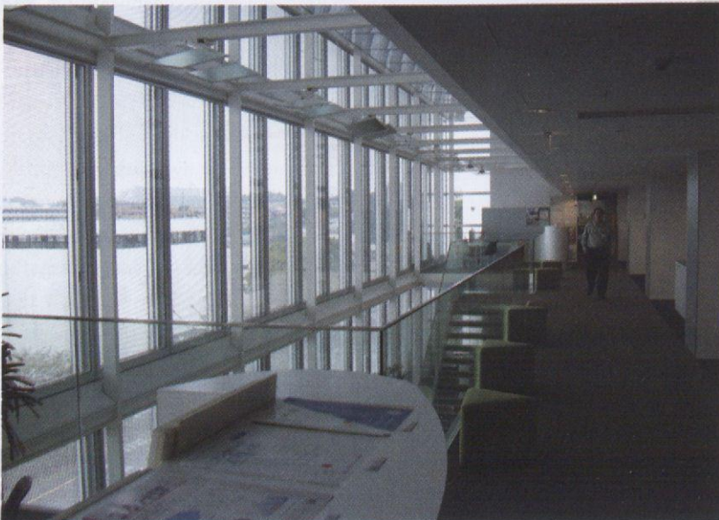
THE COMPACT DOUBLE-SCREEN IS A WINDOW SYSTEM THAT DECREASES SOLAR RADIATION HEAT. OPENING AND CLOSING THE ISOLATION DAMPERS CONTROLS THE AIRFLOW AND MAXIMIZE ENERGY SAVINGS.
