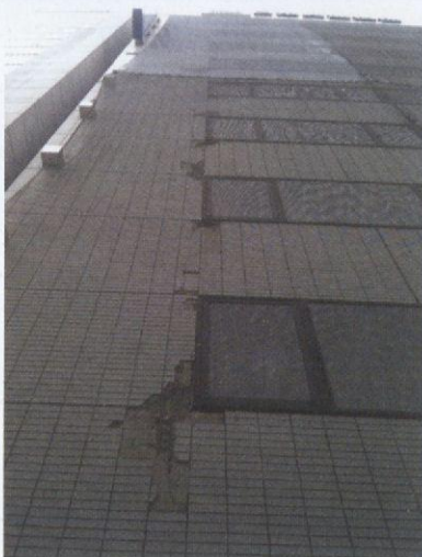
[BOTTOM] YOKOHAMA OFFICE BUILDING DAMAGE CAUSED CRACKS IN THE WALL.
